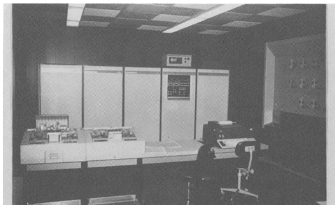
FIG. 24. View of refinery process computer and graphic panel.
